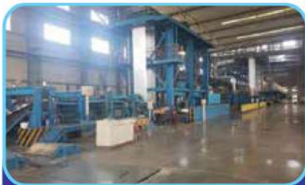
Continuous Galvanizing Line (CGL)
