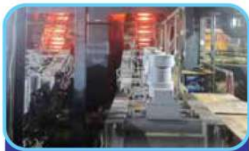
Tension Levellers in Segment
