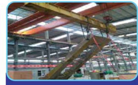
Housing of Cold Rolling Mill
