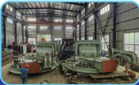
Roof of the EAF Furnace
